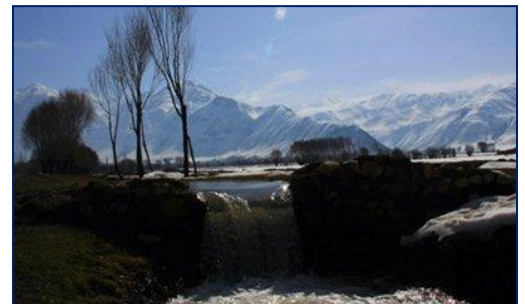
The German development corporation GIZ is bringing electricity to the remote Badakhshan and Takhar provinces in Afghanistan by constructing new off-grid hydro schemes. Photograph: Ashden Awards 2012
