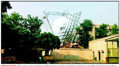
BRIGHT IDEA: The solar concentrator at the temple produces steam which powers the cooking procedure
