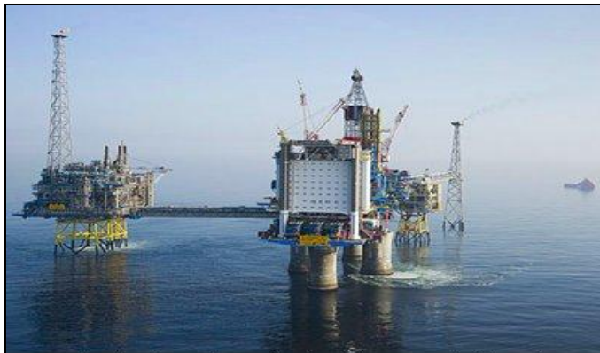
Norway's Utsira formation, under the Sleipner Gas Field, was host to the world's first commercial carbon storage project. One million metric tonnes of carbon dioxide have been injected into the undersea reservoir every year since 1996. (Photo: Oyvind Hagen / Statoil)
