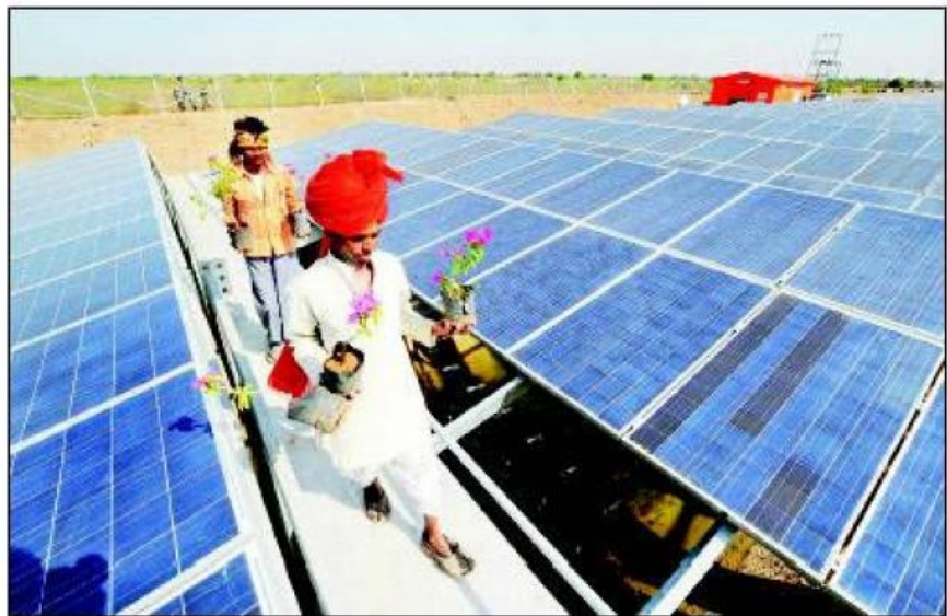
BLOOMING PLANT A worker at India's first 1MW canal-top solar power installation at Chandrasan village near Mehsana, 45 km from Ahmedabad
